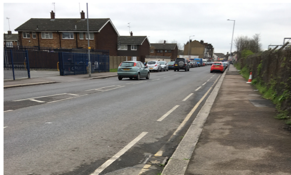
Figure 29: Existing sub-standard infrastructure along Dock Road
