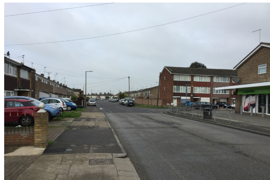
Figure 32: Lack of cycling infrastructure on Calcutta Road
